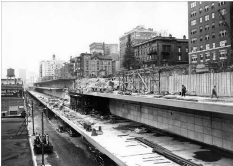
BQE Triple Cantilever construction, early 1950s. Credit: NYC DOT.
