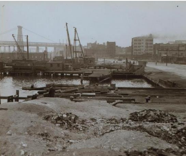
Piers and buildings on East River shoreline prior to demolition and fill for East River Park – 1937
