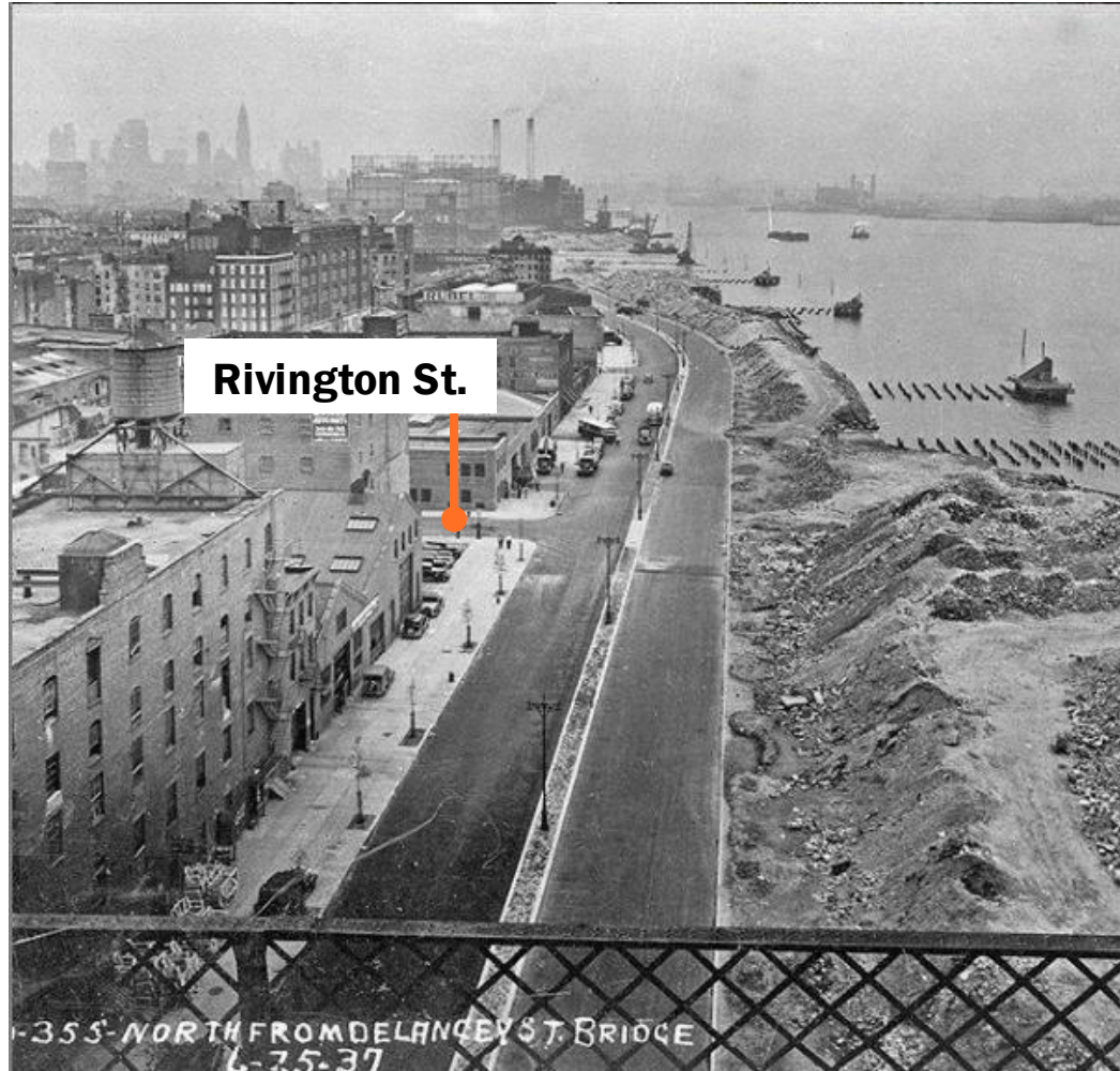
Construction of FDR Drive and East River Park infill - 1937
