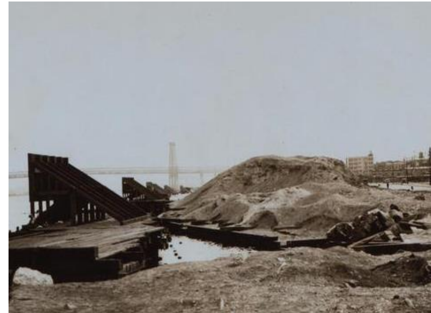
Bulkheads and pier stumps during demolition and fill for East River Park and East River Drive – 1937
