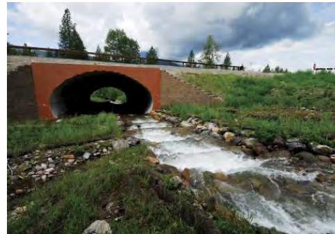
Expanded Culvert with Aquatics
