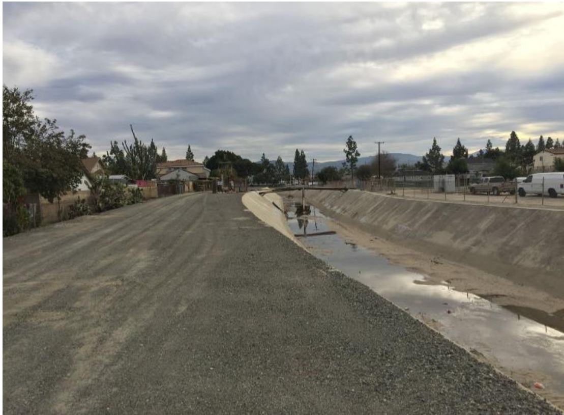
Atwood Flood Control Channel, Atwood, CA
