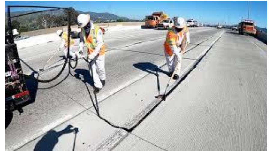
Caltrans Road Maintenance
